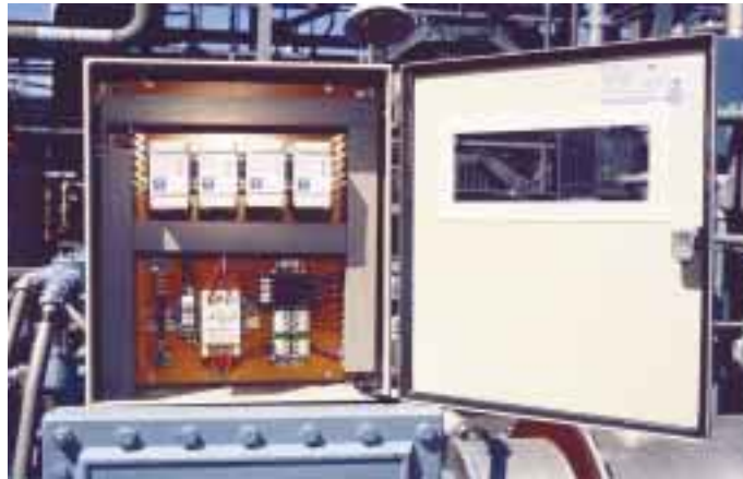
Electronic cabinet with built-in MCM™ units
